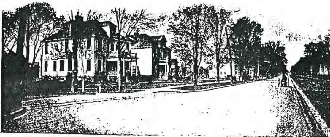
South on Genesee Street, from Proctor Boulevard
